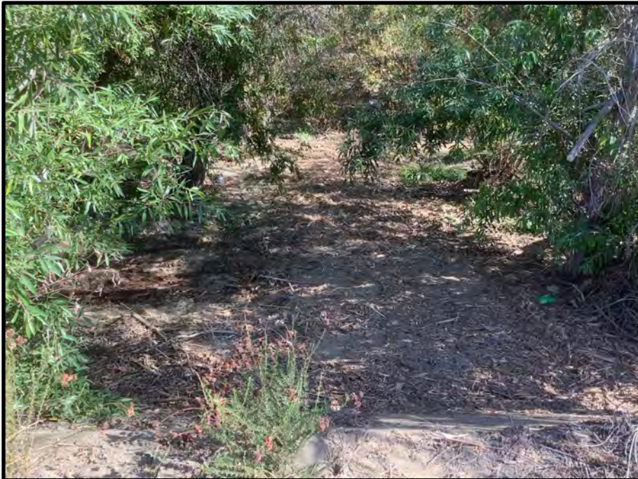
← SAWA's Green Climber LV 600 masticating blockages in the channel 11/7/23.
