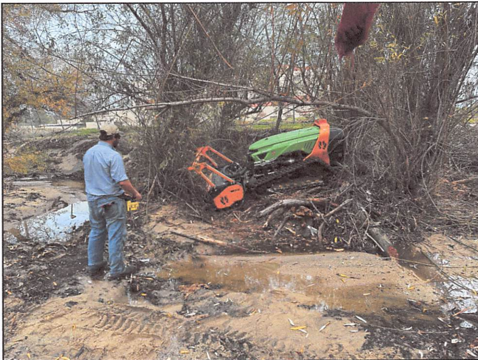
← SAWA's Green Climber LV 600 masticating blockages in the channel 12/29/22.
